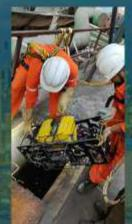
Since commissioning, inspection was not performed due to lack of shutdown (pumps running 24x7). Unmanned ROV inspection was preferred due to confined region, safer option & limited operational window. 25+ defects were identified along with construction debris that could choke the pumps
